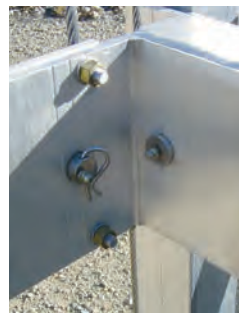
Stainless Pins with Grease Zerks
